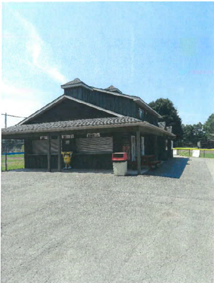
Concession Stand- Location of Restrooms and storage. Inadequate for current needs
